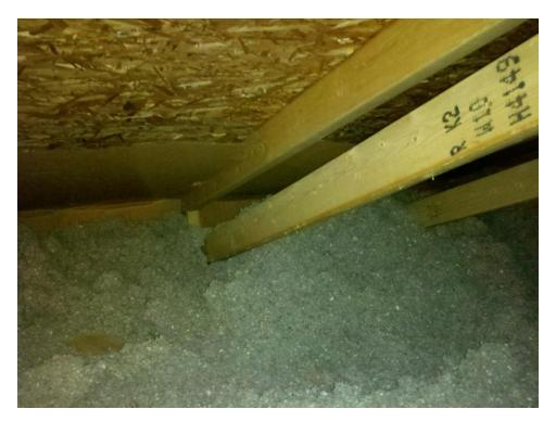
Cardboard baffle was moved to proper rafter to ensure top plate was insulated fully
