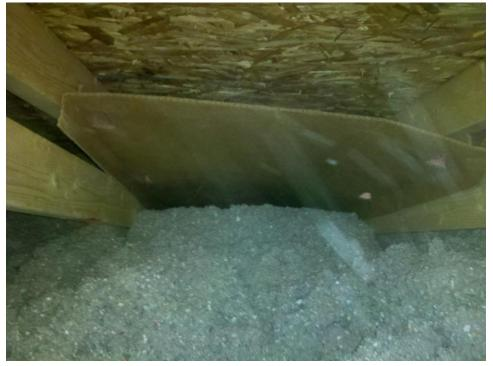
Installed Cardboard Baffle was attached to the lower of the two rafters, creating a large airspace, reducing the insulation levels over the exterior walls.
